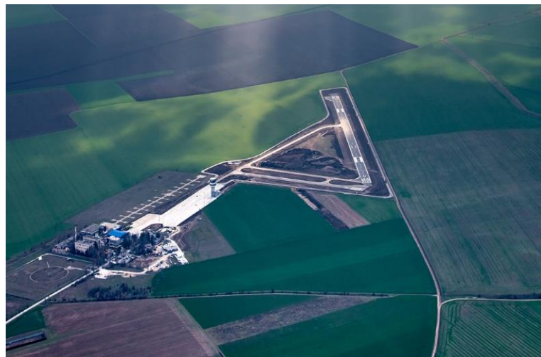
FIG. 2 Current infrastructure of Tuzla Aerodrome (Source: RAS Tuzla) [2]
